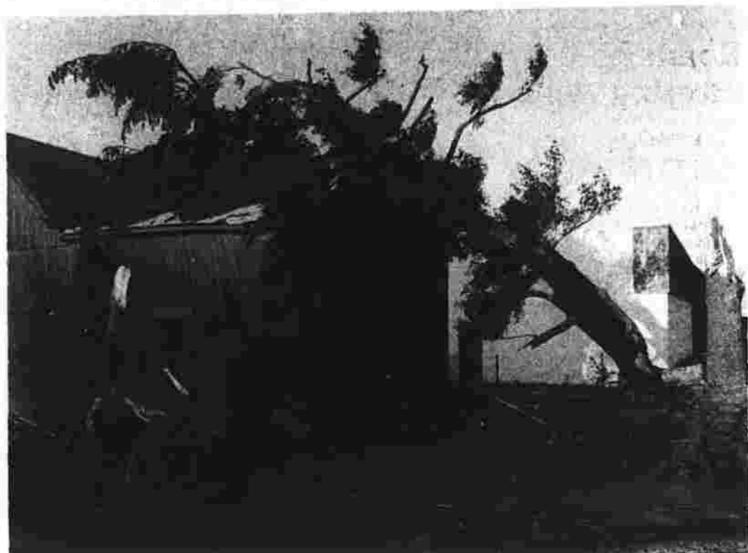
High winds Friday night caused damage of N. Charles Boggnini. (Herald photo by Adamson) was blown down at 52 Spencer St. at the home
